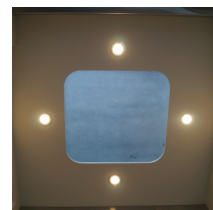
Skylight with LED Lights
