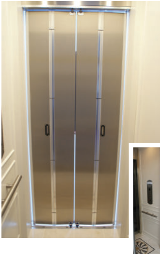
Automatic Bifold View from inside elevator
