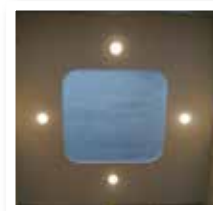
Skylight with LED Lights
