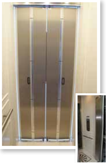
Automatic Bifold Gate View from inside elevator
