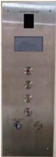
Car Operating Panel located inside the cab
