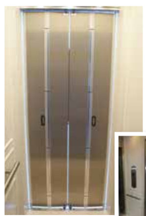
Bifold View from inside elevator
